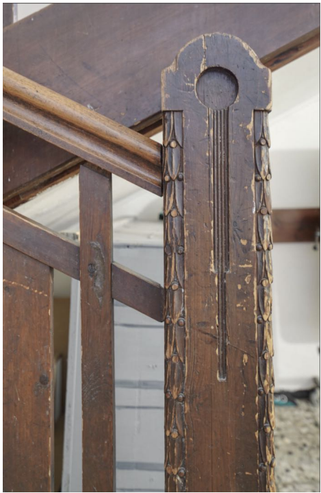
Treppe 2 - Detail Antrittsposten
